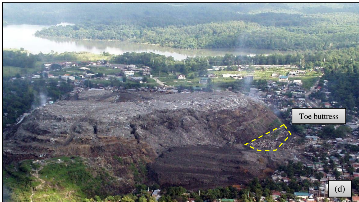
Figure 6. Slope geometry and failure surface after failure (a) evidence of seeping leachate, (b) representative slope inclination, (c) location of slope benches, (d) toe buttress (photos by S.M. Merry).
