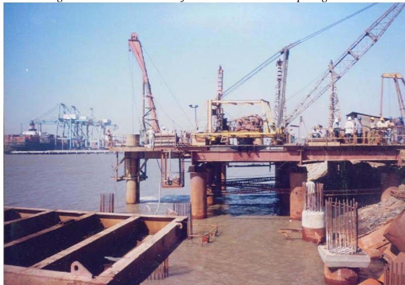
Figure 11. Construction of Piles.
