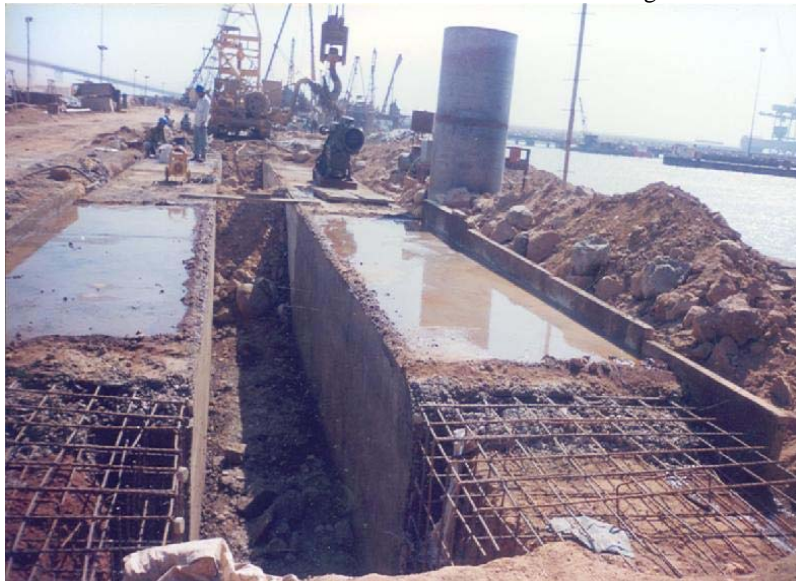
Figure 10. Construction Of Guide Walls For Diaphragm Wall.
